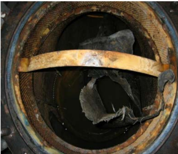
Gambar 4. Vacuum pump (LNG/C Golar Mazo document)
